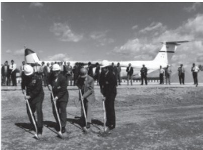
Ground breaking at Stewart International Airport in preparation for construction of the 105th Airlift Wing.
